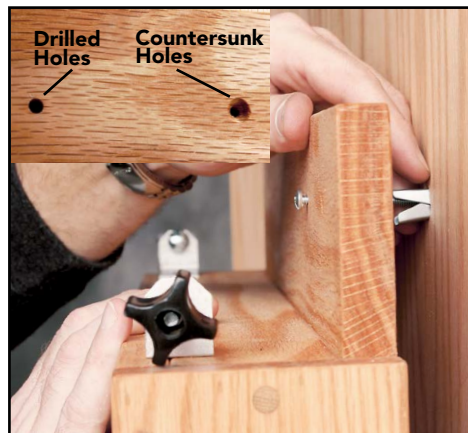
2. Insert bolts with toggles into holes drilled through wall if not screwing frame directly to studs.
