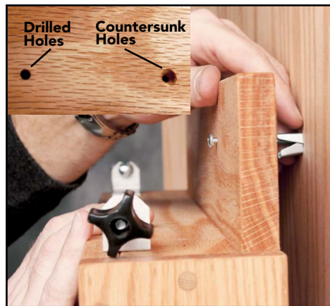
2. Insert bolts with toggles into holes drilled through wall if not screwing frame directly to studs.
